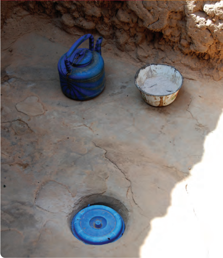
A toilet in Mali, including a covered latrine hole and a container with water.
