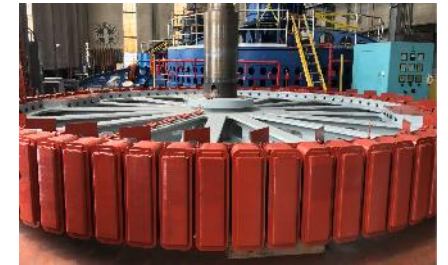
Installation of Coils on Unit #1 Rotor
